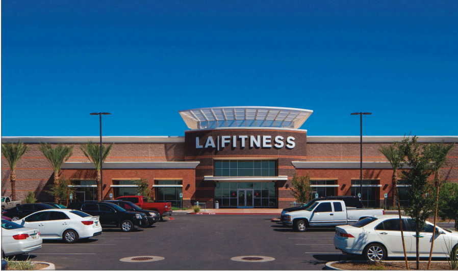
LA Fitness opened a new, 45,000-square-foot location at Rivulon in April 2015.
